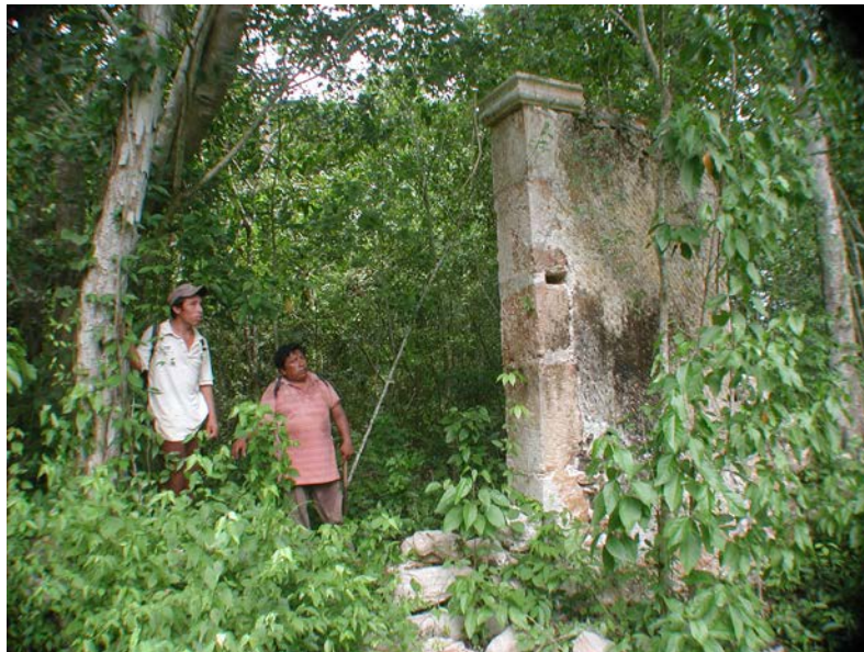
Figure 97. Photo of Wall including Cut Stones at Ramonal Poniente
