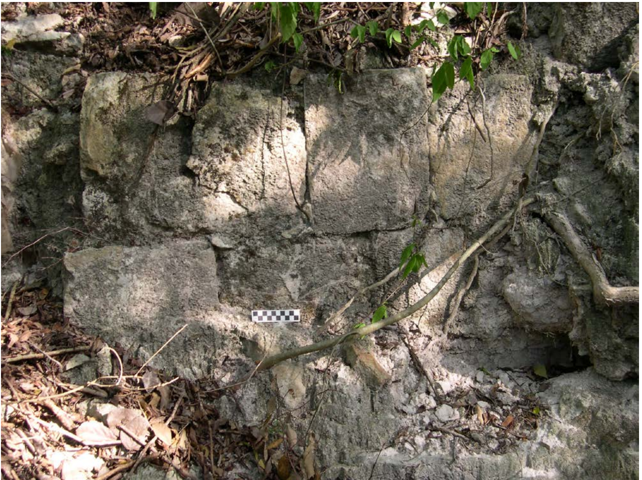
Figure 37. Photo of Construction Detail at Calotmul
