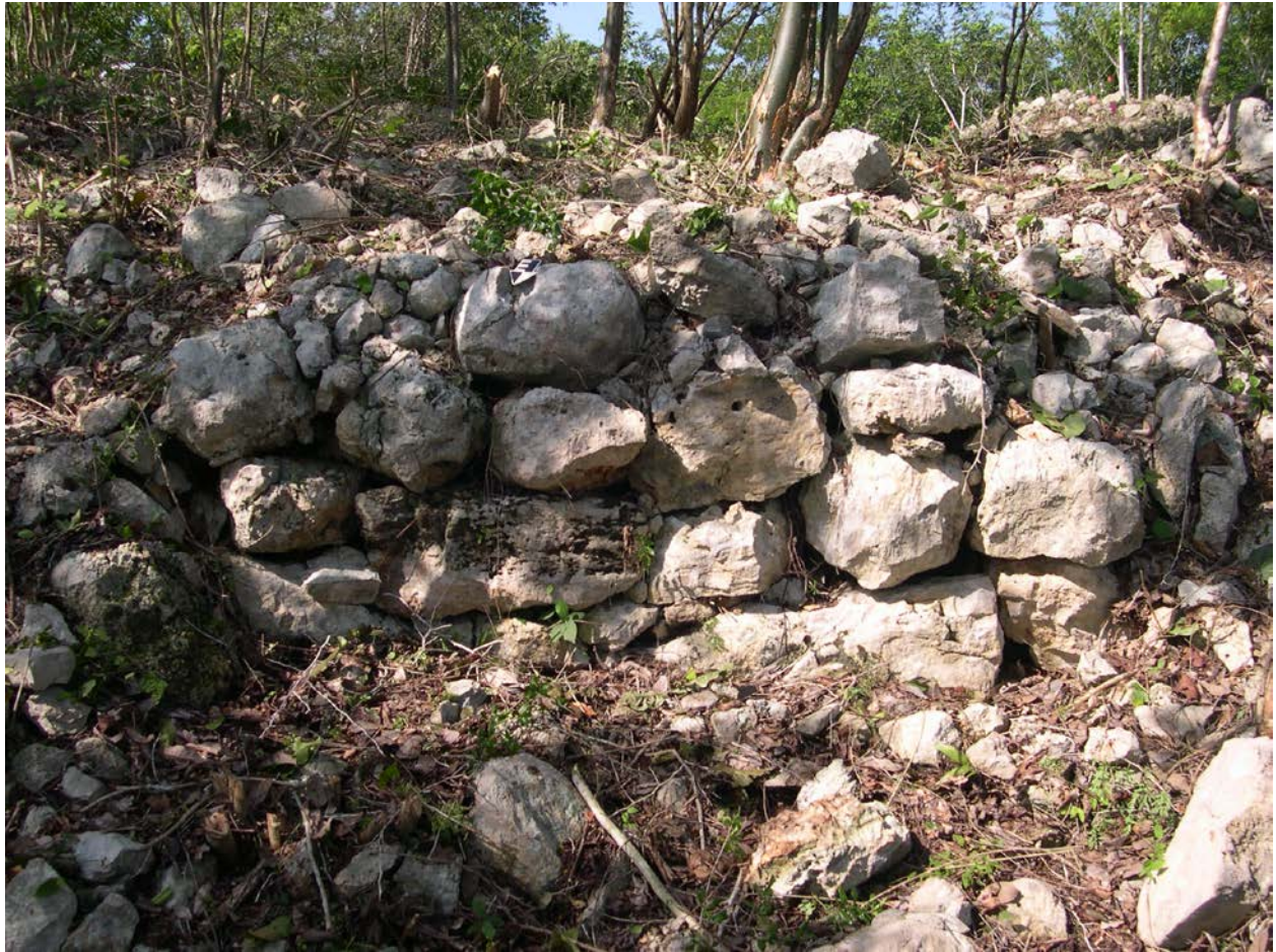
Figure 60. Structure S1W3-1 Platform Edge
