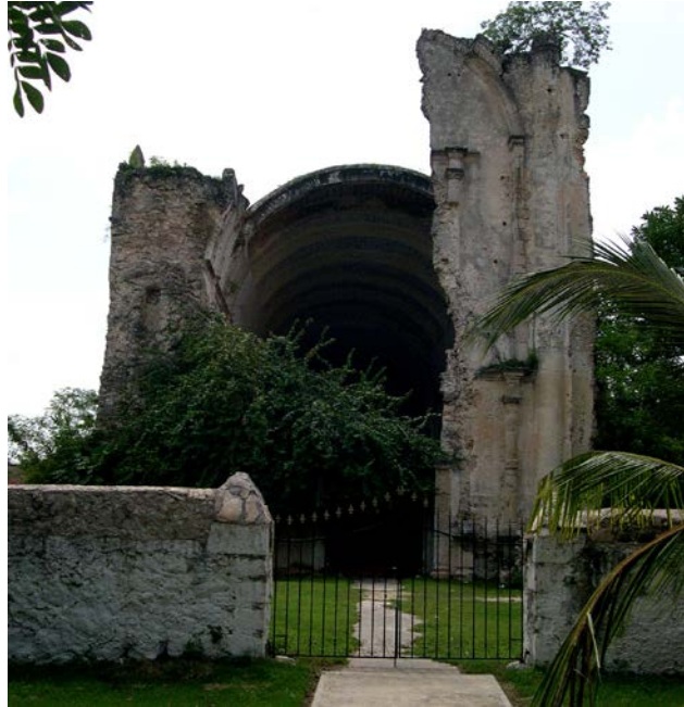
Figure 85. Photo of the Façade of the Church at Tihosuco
