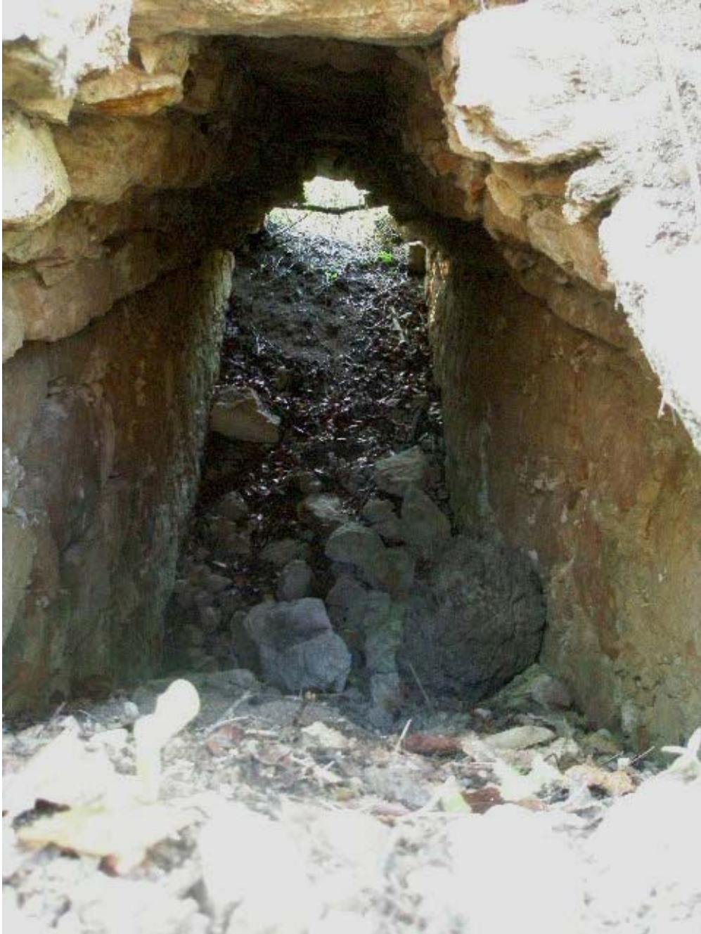
Figure 15. Vaulted Passage, Interior View
