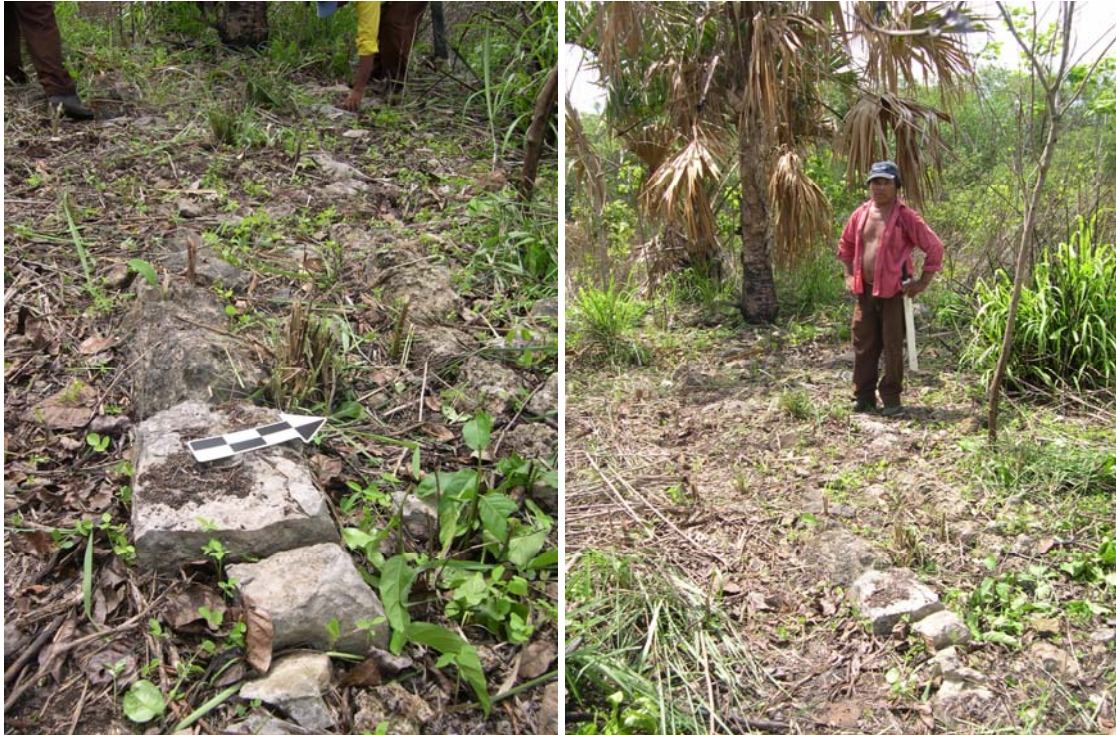
Figure 82. Rancho La Esperanza, Structure 3, Foundation Brace (southeast and western views)
