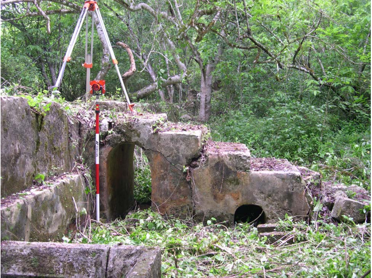
Figure 52. Xbaquil Stairs, Aqueduct, and Bebedero
