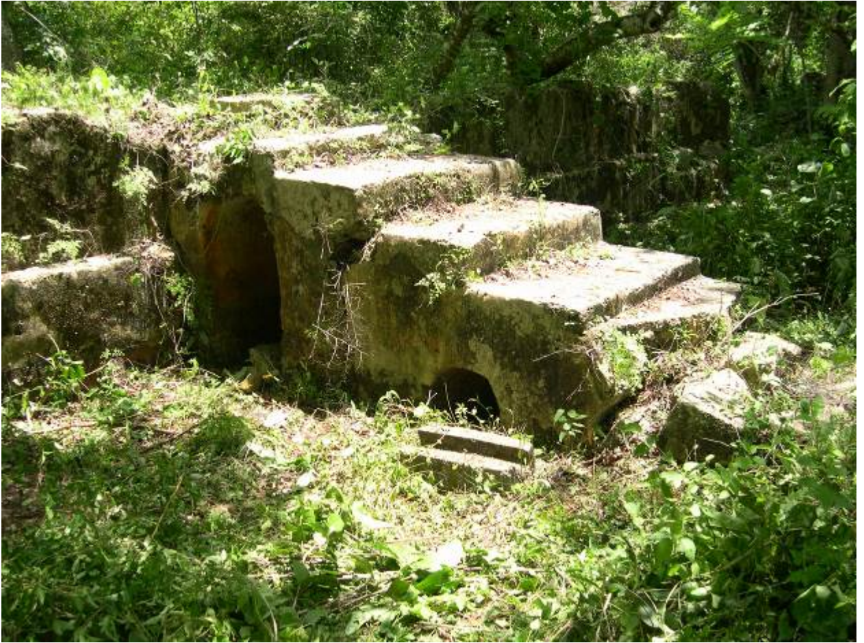
Figure 41. East View of the First Stairway
