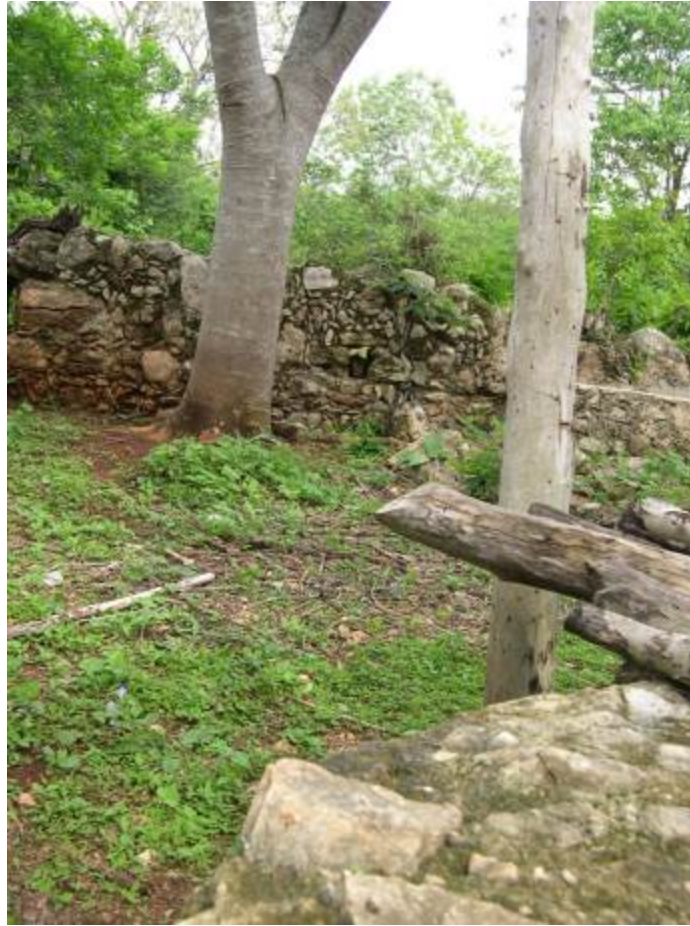
Figure 55. Detail of Colonial Wall, Viewed from the Well
