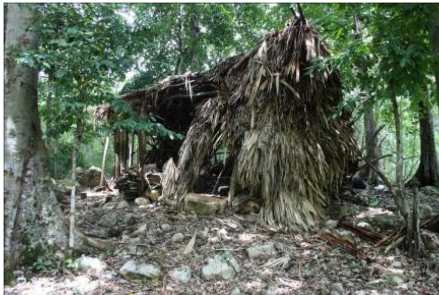
Figure 58. Top of Structure S1E1-1
