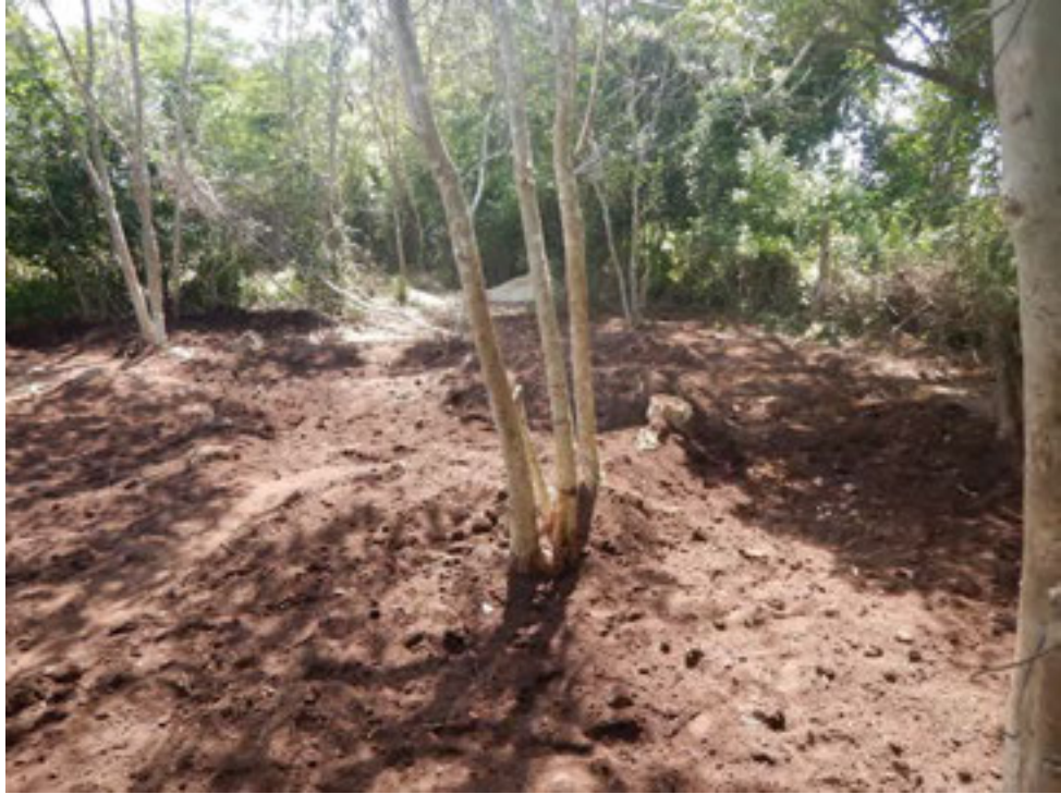
Figure 242. Sisal, Operation 8, Backfilled
