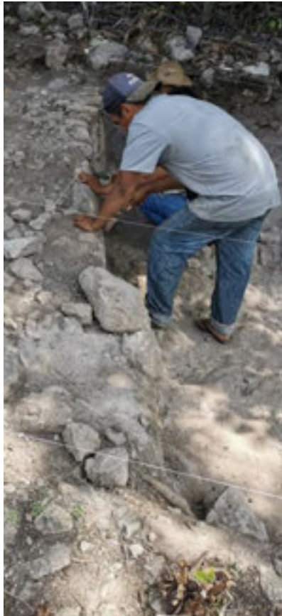
Figure 213. Operation 20, Consolidation Process
