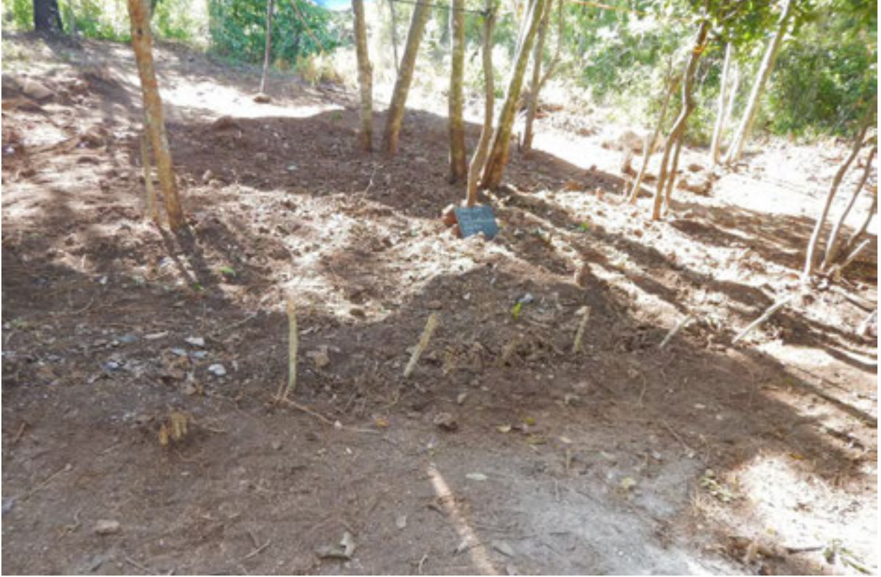
Figure 311. Sisal, Operation 9, Backfilled
