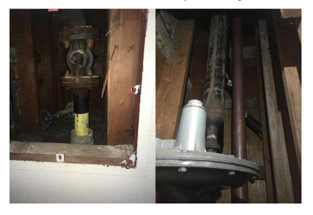
N. Picture 23 shows all the drinking fountain hose bib shut off valves and clean out. All of this is to be abated. Note, 12KV lines are underground in the breezeway between Life Science and Physical Science – likely less than 3 feet below grade – USE CAUTION.
